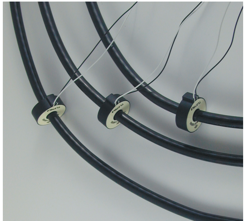
Current Transformer Alignment
