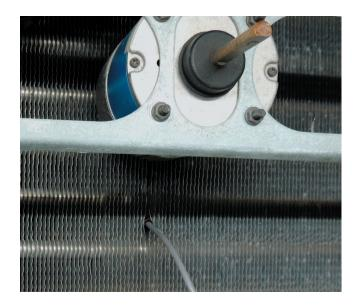
3a. Connect the Evaporator Coil Ice Sensor to terminals ICE1& GND per the wiring diagram on Page 7.
