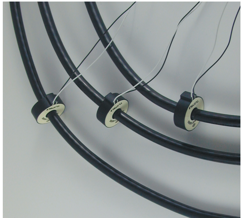
Current Transformer Alignment Figure 1
